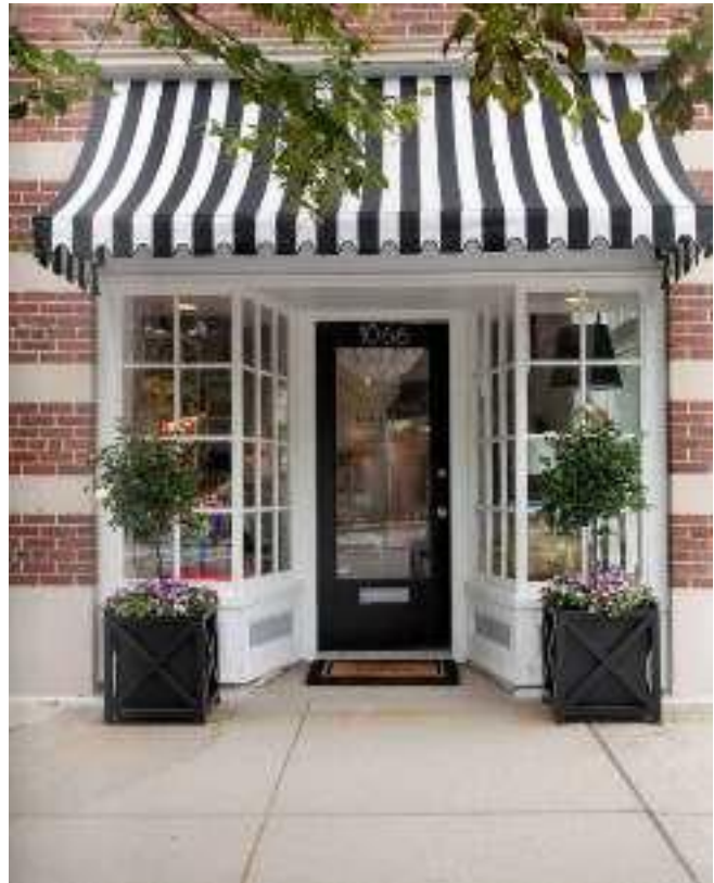
Example of primary entrance
