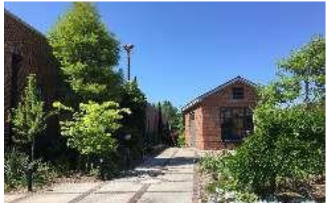
Example of sloped area with plantings
