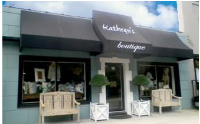
Canopy articulating main entry
