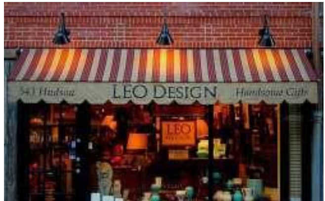
Lighting attached to facade illuminating canopy
