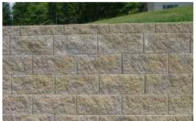
Example of split-faced masonry wall
