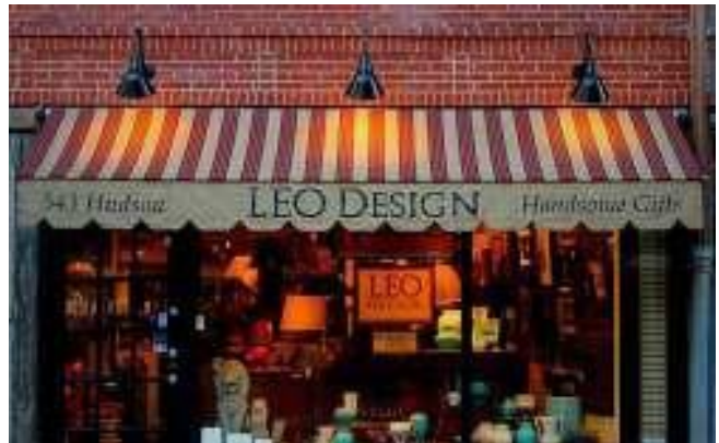
Lighting attached to facade illuminating canopy
