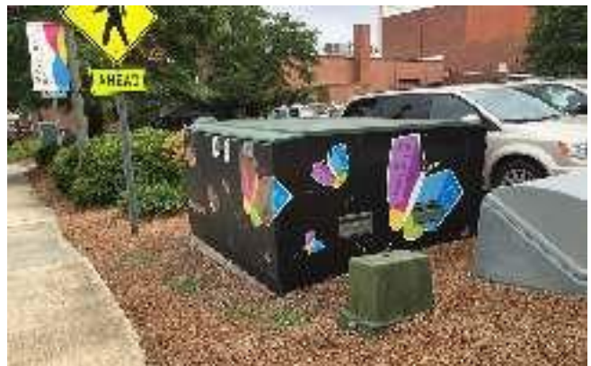
Example of trash storage area
